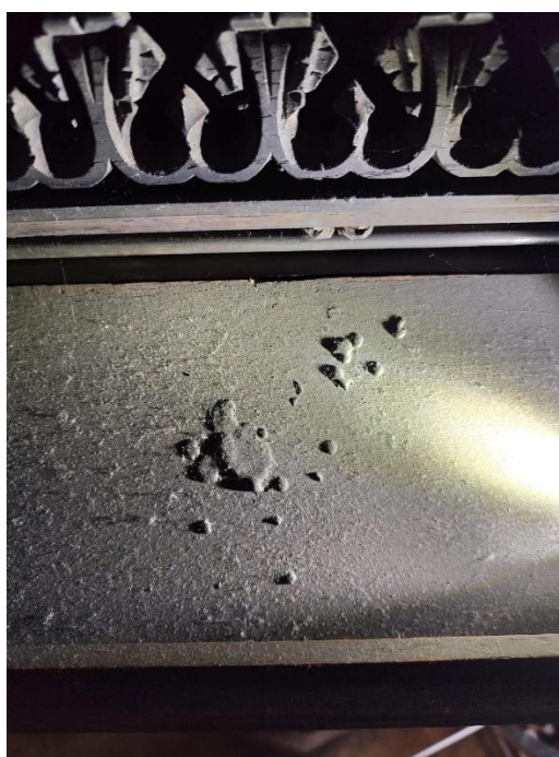
Figure 16 shows the drops of a resinous material on the canopy.
