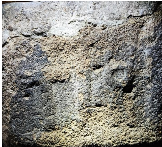
Figure 8 Diffuse abrasion and loss caused the loss of details across this carved panel.
