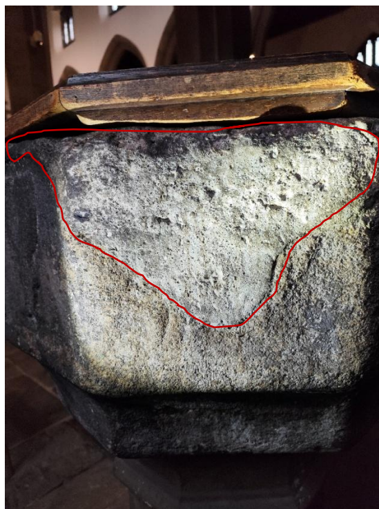
Figure 5 show the mortar repair on the east side of the font, highlighted in red.
