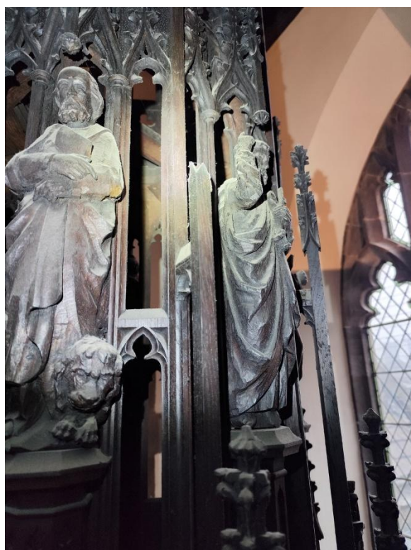
Figure 18 show missing pinnacle on the carved woodwork.
