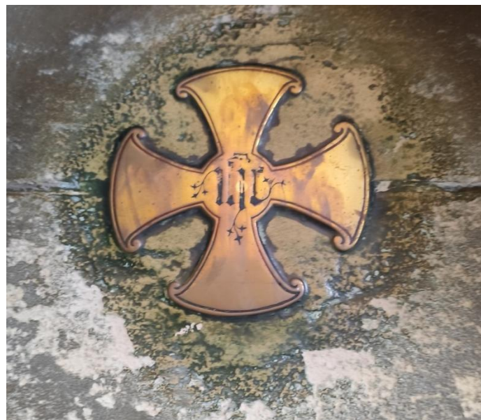
Figure 34 show the polished area of the stone adjacent to the cross, suggesting the use of abrasive cleaning.
