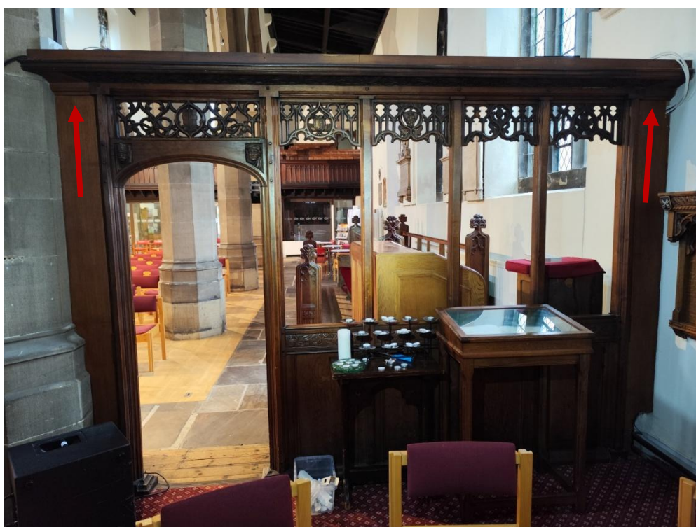
Figure 25 show the suggested lifting points.
