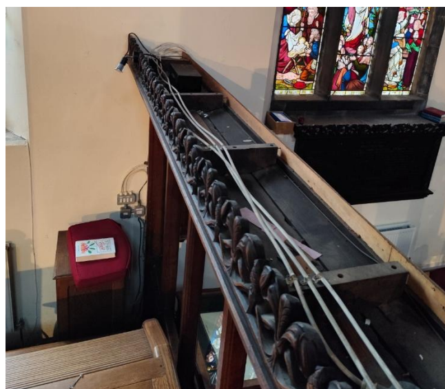
Figure 22 it shows the cables on the upper section of the memorial.
