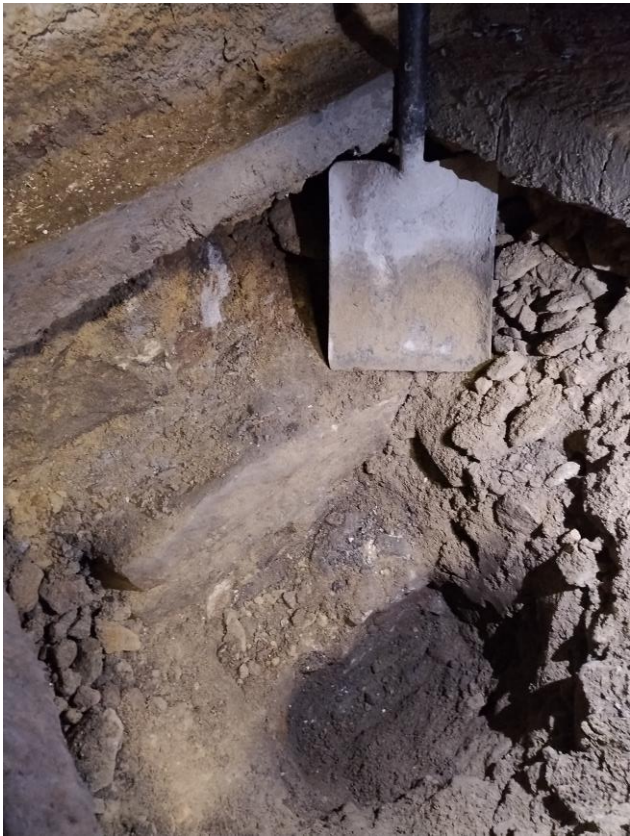
Photo 1 – General view on trial hole showing excavation and outstand of stone footing and lime mortar mix concrete.
