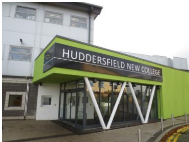
Huddersfield New College Main Entrance Extension
