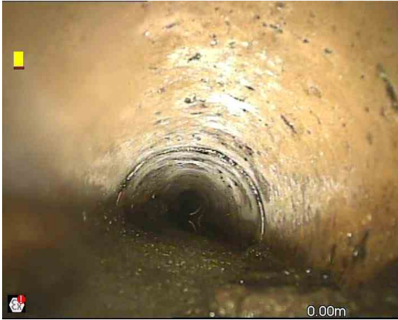
HOLX_f5b15a02-15c6-49ca-ad68-5e1ce1ecfc98_20241204_093814_295.jpg, 00:00:03, 0.00 m Settled deposits, fine, 25% cross-sectional area loss, start
