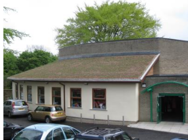
Shelf Village Hall, Halifax Library Extension
