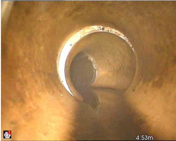
MH4X_25a2e17d-f70c-44fa-9597-381f4a33c61e_20241204_1 00732_816.jpg, 00:00:25, 4.80 m Joint displaced, medium
