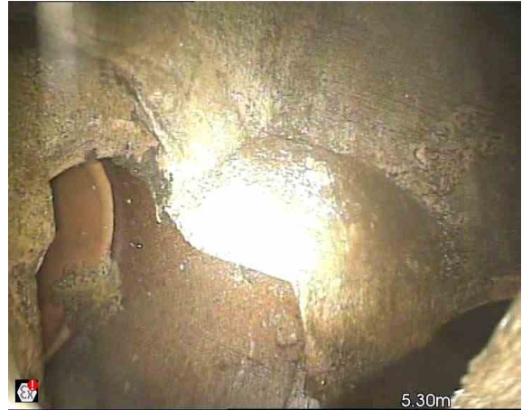
MH4X_d37e2720-9af4-4fd0-a4cf-d79205e8e24a_20241204_1 00757_651.jpg, 00:00:29, 5.30 m Finish node, manhole, reference: Discharge, Manhole-5
