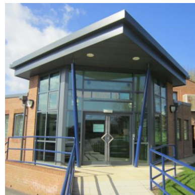
St Mary's High School, Chesterfield Main Entrance Extension
