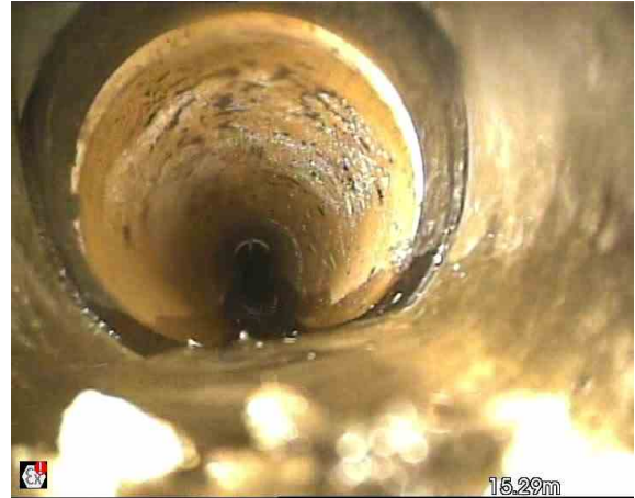
HOLX_35a4a035-aa73-40cb-916c-0bc3d1fdb085_20241204_093653_793.jpg, 00:00:52, 15.20 m Finish node, manhole, reference: HOL, Manhole-3
