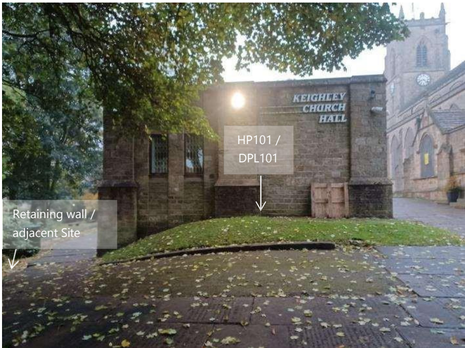
Photograph 2: View from the eastern portion of the Site looking west towards the existing church hall
