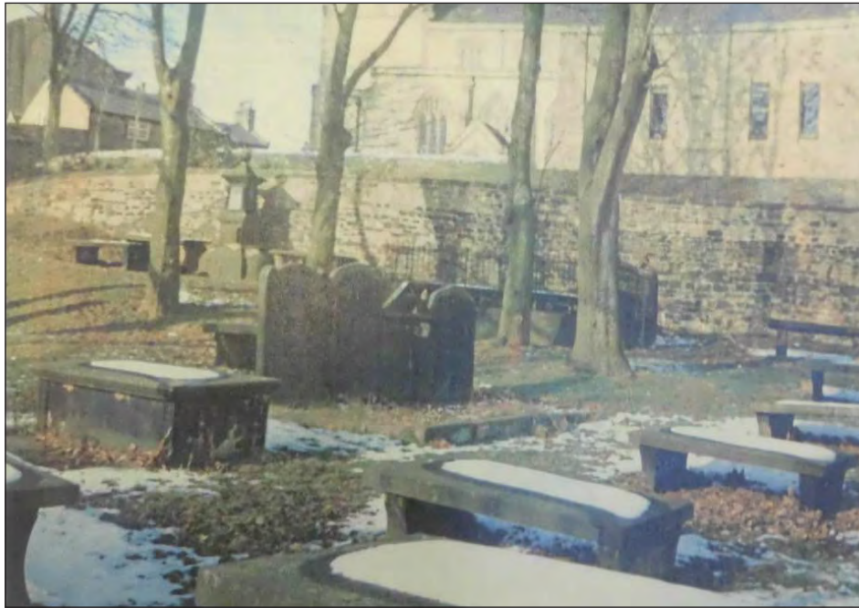
Plate 7. View of Church and retaining wall before 1982, looking north
