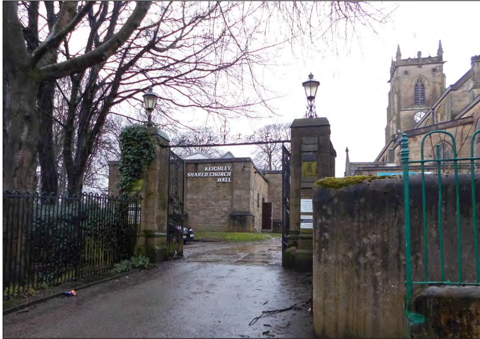
Plate 1. View of the church hall from Market Sreet, looking west
