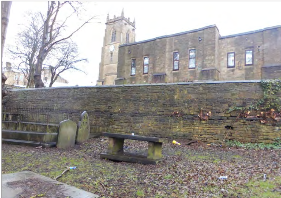
Plate 5. View of the church hall and retaining wall from graveyard, looking north
