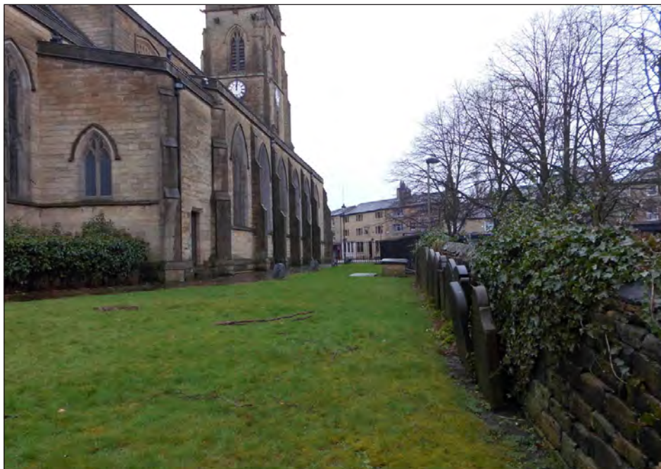
Plate 6. View of graveyard to the north of the Church, looking west
