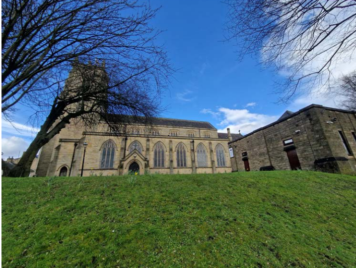
View from South looking towards Southern Elevation of the parish church and former methodist hall building
