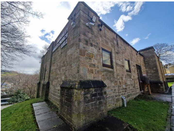
View of North East Corner of former methodist hall building
