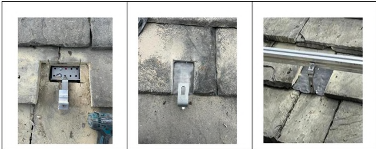
Installation stages on a Yorkshire stone roof.
