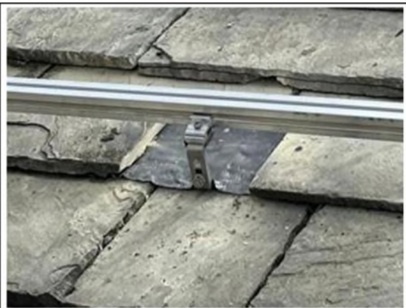
Lead dressed hook and rail installation
