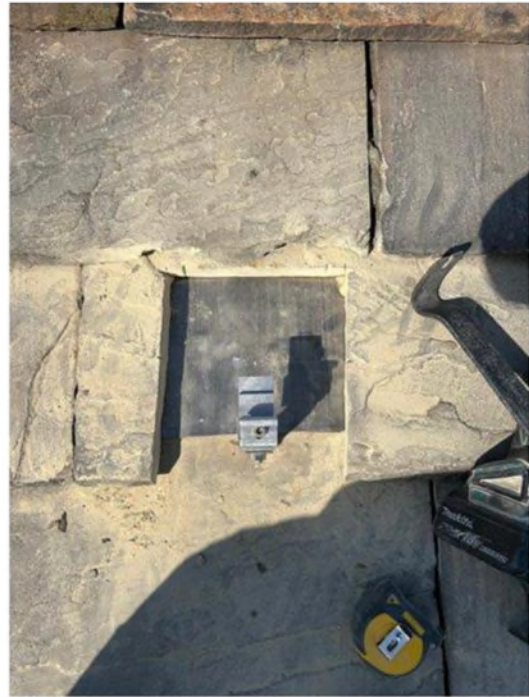
Lead flashing around hook for watertight seal
