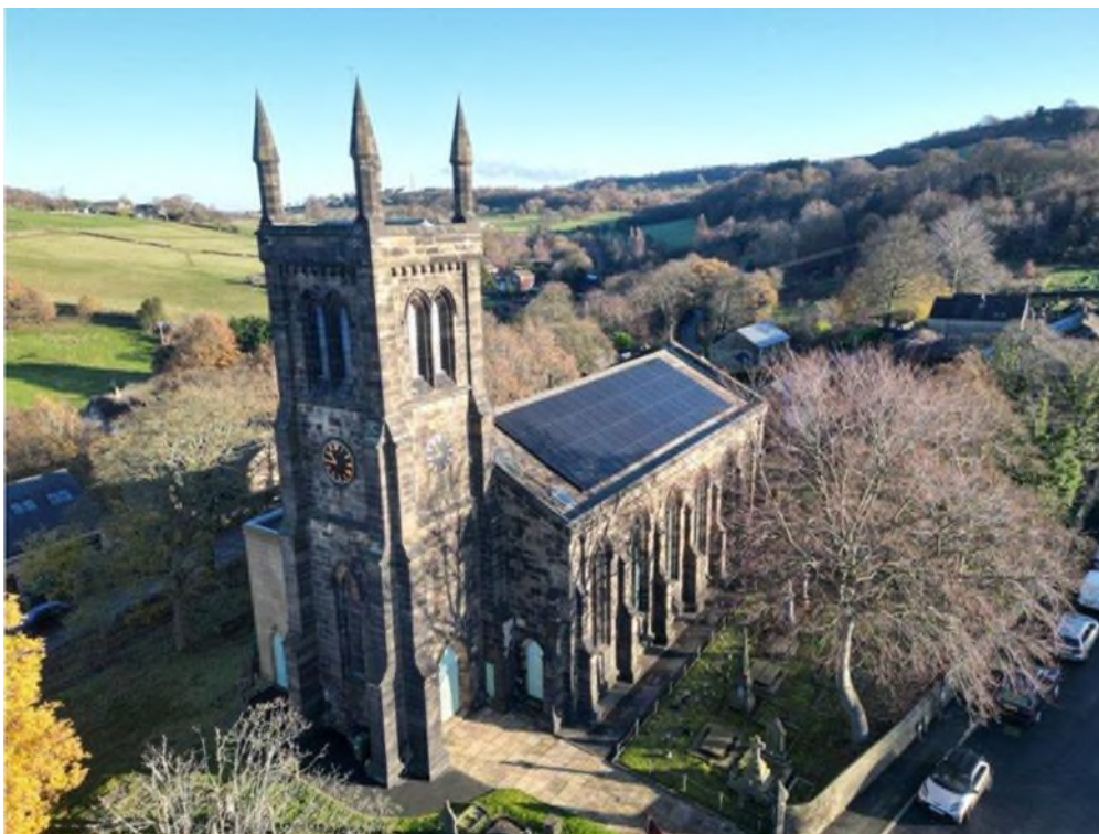
Aerial view of the completed New Mill Church installation, demonstrating the clean, professional finish achieved on a stone slate roof.
