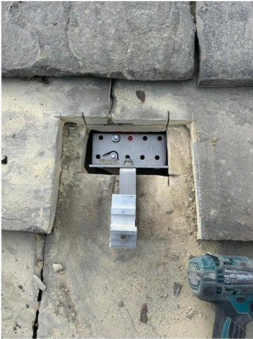
Stone roof hook installation detail
