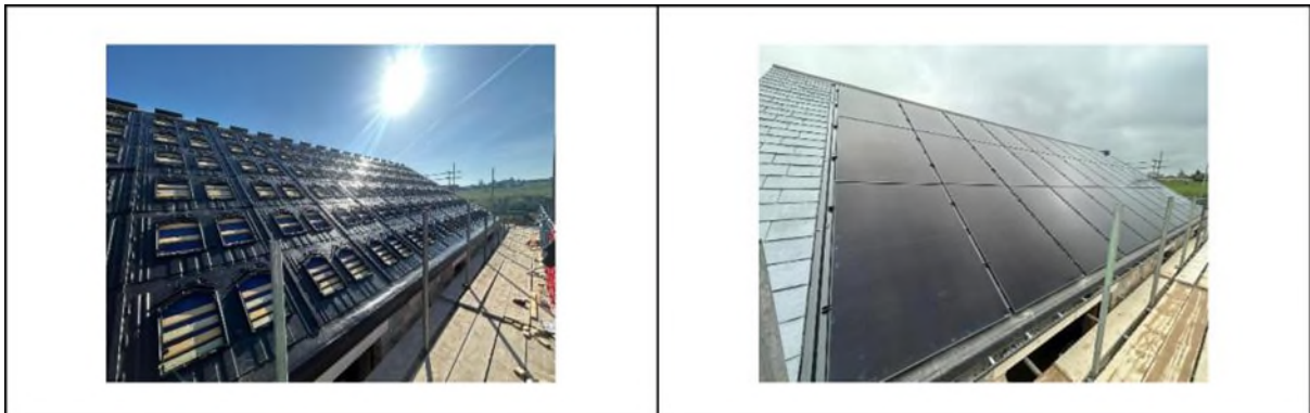
Main installation stages using GSE in roof frames.
