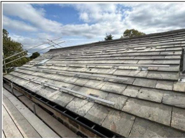
Hook and rail system on stone roof
