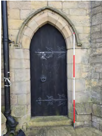
55. MC North Facing Elevation Middle Section General Shot (Bay 8) Door Shot South | 1x2
