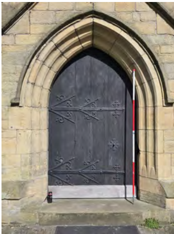
87. MC South Facing Elevation General Shot (Bay 4) Door Detail North | 1x2
