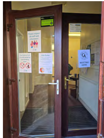
28. Community Hall (CH) North Facing Elevation (Left Hand Side (LHS)) North | 1x2
