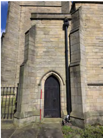
81. MC South Facing Elevation General Shot (Bay 1) Corner Shot North | No Scale
