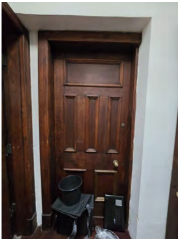
213. G13 North Wall Door North | No Scale
