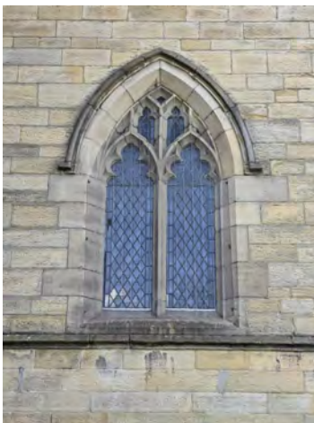
41. MC East Facing Elevation (RHS) Window Detail Shot East | No Scale
