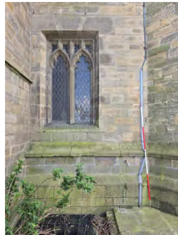
58. MC East Facing Elevation General Shot (Bay 9) Ground Floor South | 1x2
