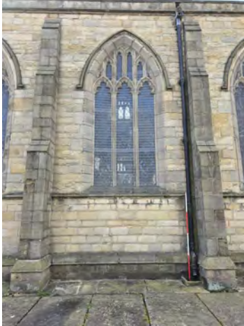
49. MC North Facing Elevation Middle Section General Shot (Bay 3) South | 1x2
