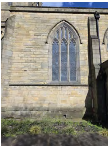
83. MC South Facing Elevation General Shot (Bay 2) Door Detail North | 1x2
