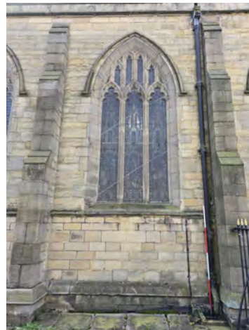
52. MC North Facing Elevation Middle Section General Shot (Bay 6) South | 1x2
