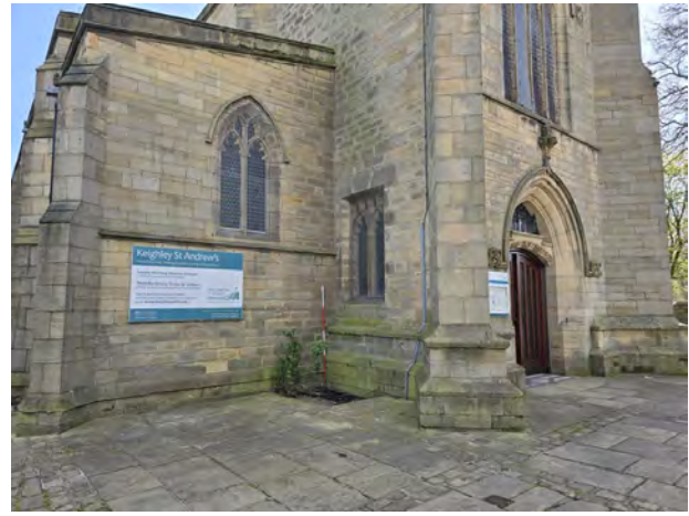
62. MC West Facing Elevation Corner Shot General Shot North | 1x2
