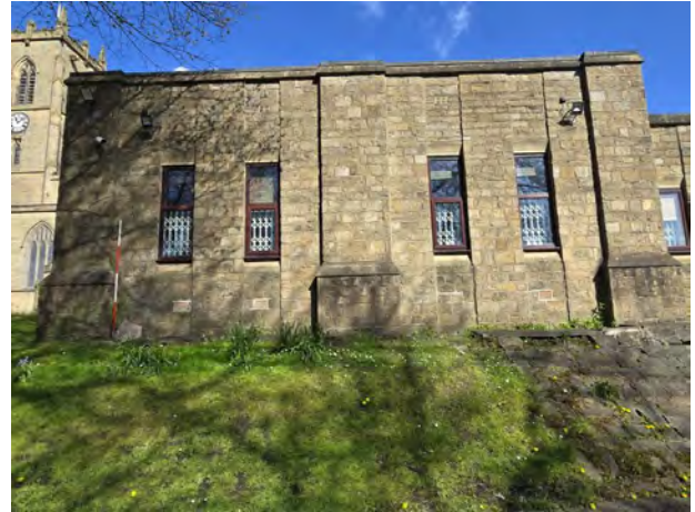
32. CH South Facing Elevation (RHS) South | 1x2
