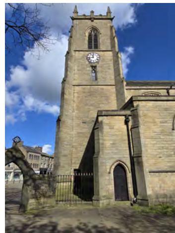
78. MC South Facing Elevation General Shot (Bay 1) Door Detail North | 1x2
