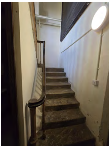
113. G4 Staircase Shot North | No Scale
