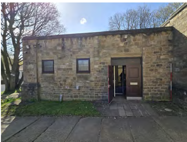
29. CH North Facing Elevation (Right Hand Side (RHS)) North | 1x2
