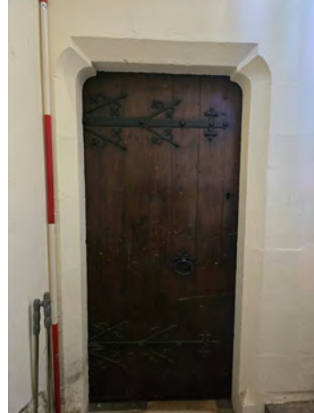
146. G6 Stair East Wall East | 1x2
