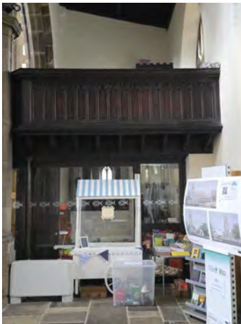
231. G7 Pew Shot West Wall Bay 1 (RHS) West | No Scale
