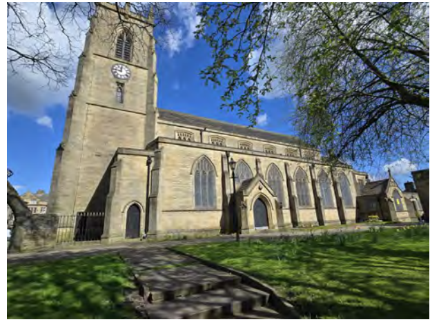
80. MC South Facing Elevation General Shot (Bay 1) First and Second Floor North | No Scale
