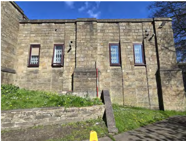
33. CH South Facing Elevation (RHS) Corner Shot North-West | No Scale
