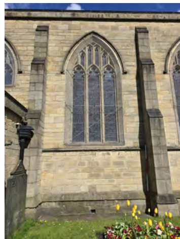
90. MC South Facing Elevation General Shot (Bay 5) North | 1x2
