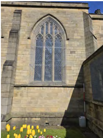
93. MC South Facing Elevation General Shot (Bay 8) North | 1x2
