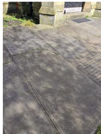
84. MC South Facing Elevation General Shot (Bay 3) North | 1x2
