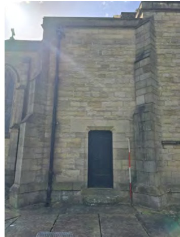
46. MC North Facing Elevation Middle Section General Shot (Bay 1) South | 1x2
