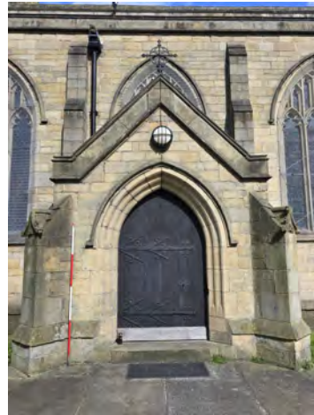
86. MC South Facing Elevation General Shot (Bay 4) Principal Elevation North | 1x2
