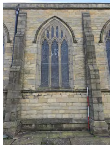
50. MC North Facing Elevation Middle Section General Shot (Bay 4) South | 1x2
