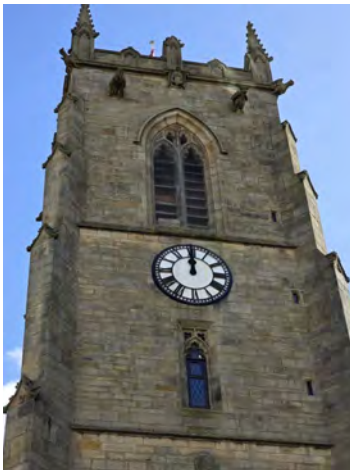
69. MC West Facing Elevation General Shot (Bay 2) First Floor South-East | No Scale
