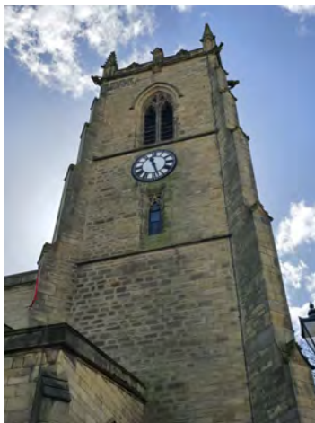
59. MC East Facing Elevation General Shot (Bay 9) First Floor South | No Scale
