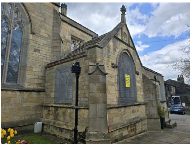
239. MC Bay 9 West Facing Elevation Corner Shot North-East | 1x2
