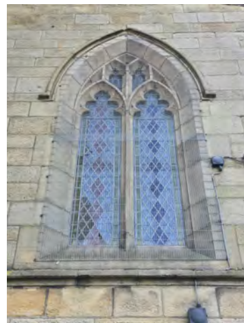
72. MC West Facing Elevation General Shot (Bay 3) Corner Shot West | 1x2
