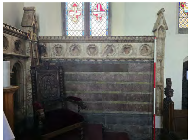
184. G10 Eastern Portion South Wall West | No Scale
