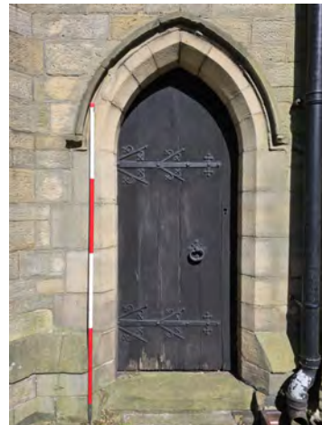
82. MC South Facing Elevation General Shot (Bay 2) North | 1x2
