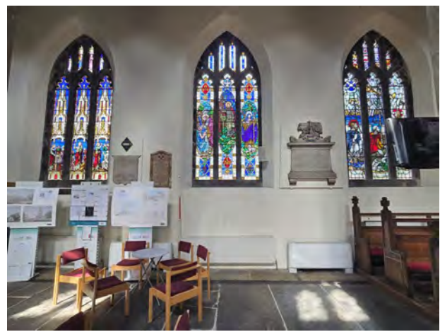
160. G7 North Wall Bays 1, 2 and 3. North | 1x2
