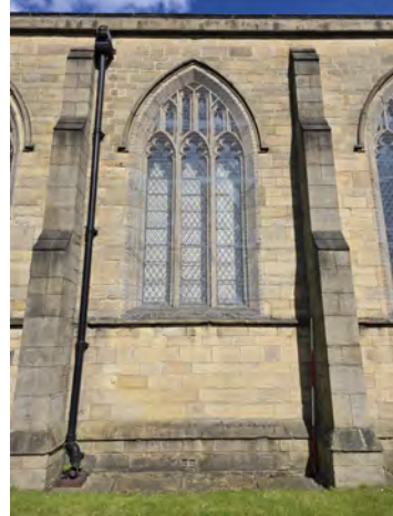
92. MC South Facing Elevation General Shot (Bay 7) North | 1x2
