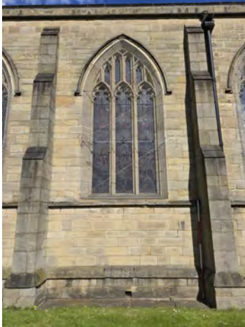
91. MC South Facing Elevation General Shot (Bay 6) North | 1x2
