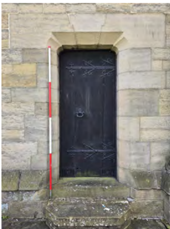
47. MC North Facing Elevation Middle Section General Shot (Bay 1) Door Detail South | 1x2
