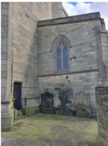
71. MC West Facing Elevation General Shot (Bay 3) South-West | 1x2
