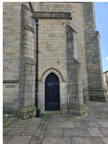
54. MC North Facing Elevation Middle Section General Shot (Bay 8) South | 1x2
