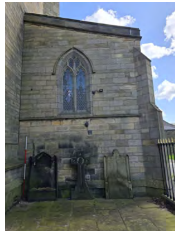
70. MC West Facing Elevation General Shot (Bay 2) Second and Third Floor South | No Scale
