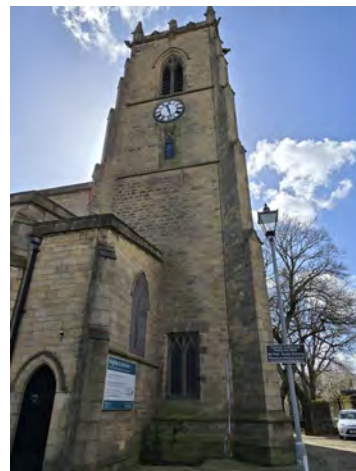
60. MC East Facing Elevation General Shot (Bay 9) General Tower Shot South | No Scale
