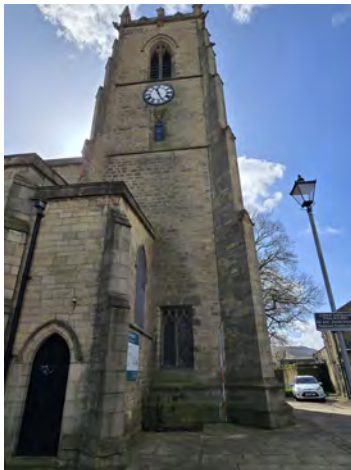
57. MC East Facing Elevation General Shot (Bay 9) South | 1x2
