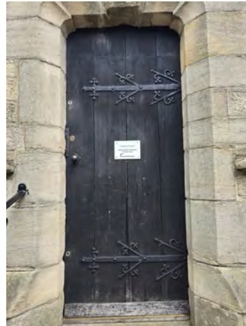
242. MC Bay 10 South Facing Elevation Door Detail North | 1x2
