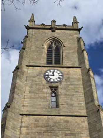
79. MC South Facing Elevation General Shot (Bay 1) General Tower Shot North | 1x2
