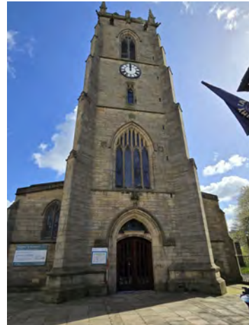
66. MC East Facing Elevation General Shot (Bay 9) Basement Detail North-West | No Scale
