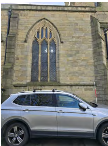
53. MC North Facing Elevation Middle Section General Shot (Bay 7) South | 1x2
