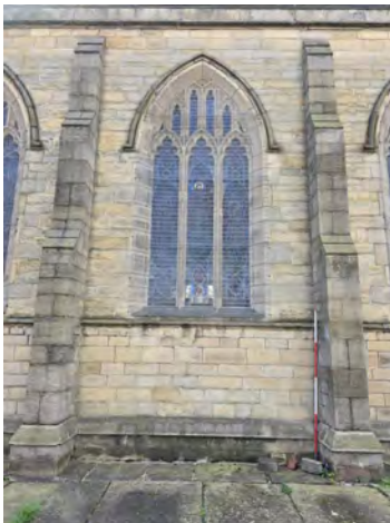
51. MC North Facing Elevation Middle Section General Shot (Bay 5) South | 1x2
