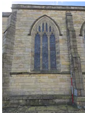
48. MC North Facing Elevation Middle Section General Shot (Bay 2) South | 1x2
