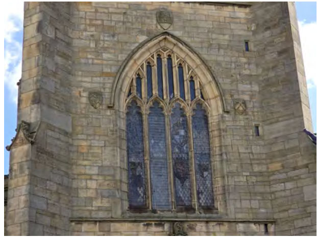
68. MC West Facing Elevation General Shot (Bay 2) Door Detail North-East | 1x2
